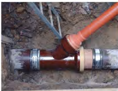
Reparatur in offener Baugrube
